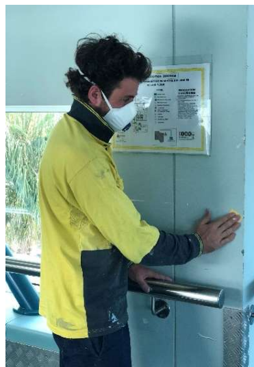
Wearing a P2 dust Masks are also required when undertaking dusty jobs such as sanding
